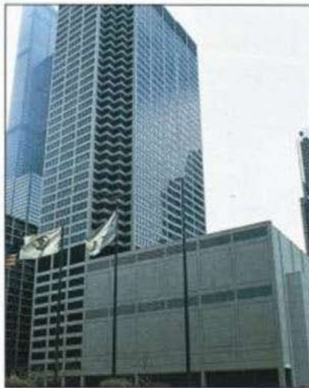
The CME building
